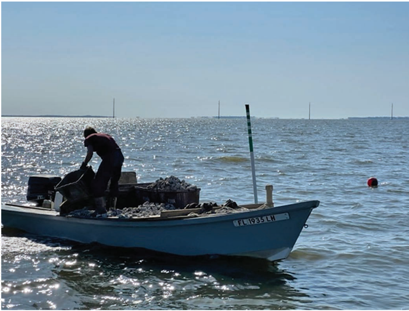
An oysterman carefully dumps concrete pieces onto one of the offshore restoration experiment sites. The green site, marked out by a 16-foot PVC pole has 12 inches of concrete pieces and 3 inches of shell on top.
