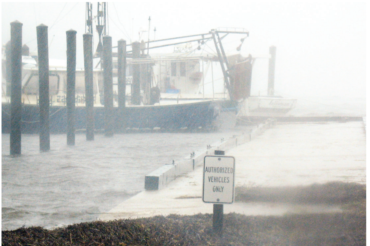
The dock in Panacea during Tropical Storm Debby.
