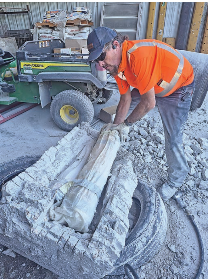
County Road and Bridge workers chiseled through some 30 inches of concrete to get to the 1976 time capsules.
